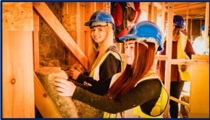
Figure 6: Valleys Kids residential Centre and Service barn, North Gower from the view of the LBG terrace Figure 7: OBF participants install sheep wool insulation in internal walls of residential centre
